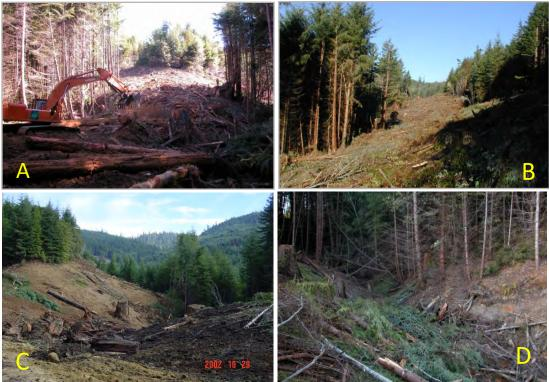
Figure 2—A. stream crossing being excavated; B. outsloped road with heavy mulching; C. recently excavated stream crossing with large woody debris placed within the exhumed channel; D. excavated stream crossing with a relatively large volume of woody debris added.
